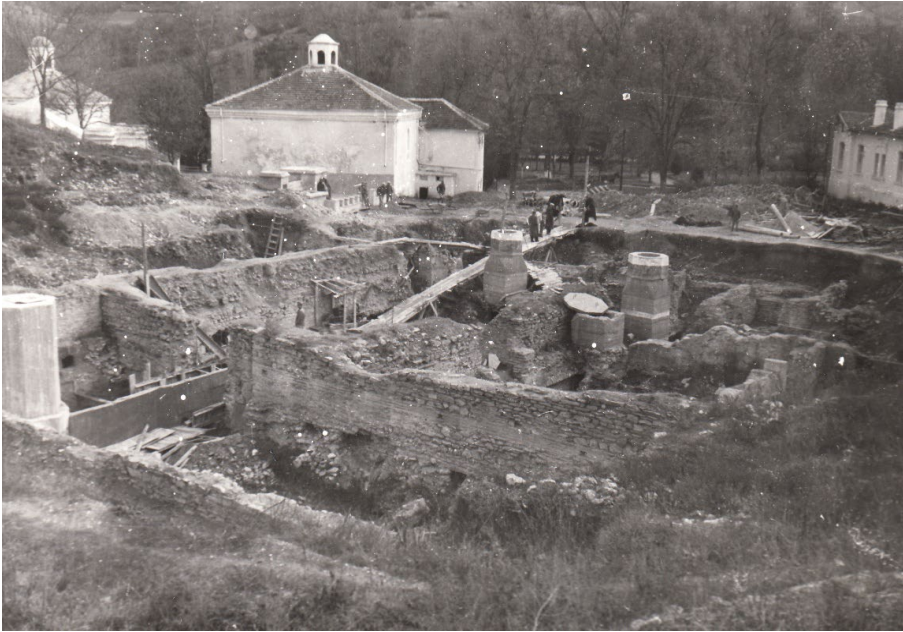
Fig. 17. Capturing of the thermal springs in Starozagorski mineralni bani in the 1950s. In the foreground are the remains of the Roman thermae ; behind them, to the left, are two Ottoman public baths. The concrete columns in the center of the image are the shafts of the captured springs, drilled right into the marble pools of the ancient thermae (NINKN, St. Z.-64-37-IVA).
